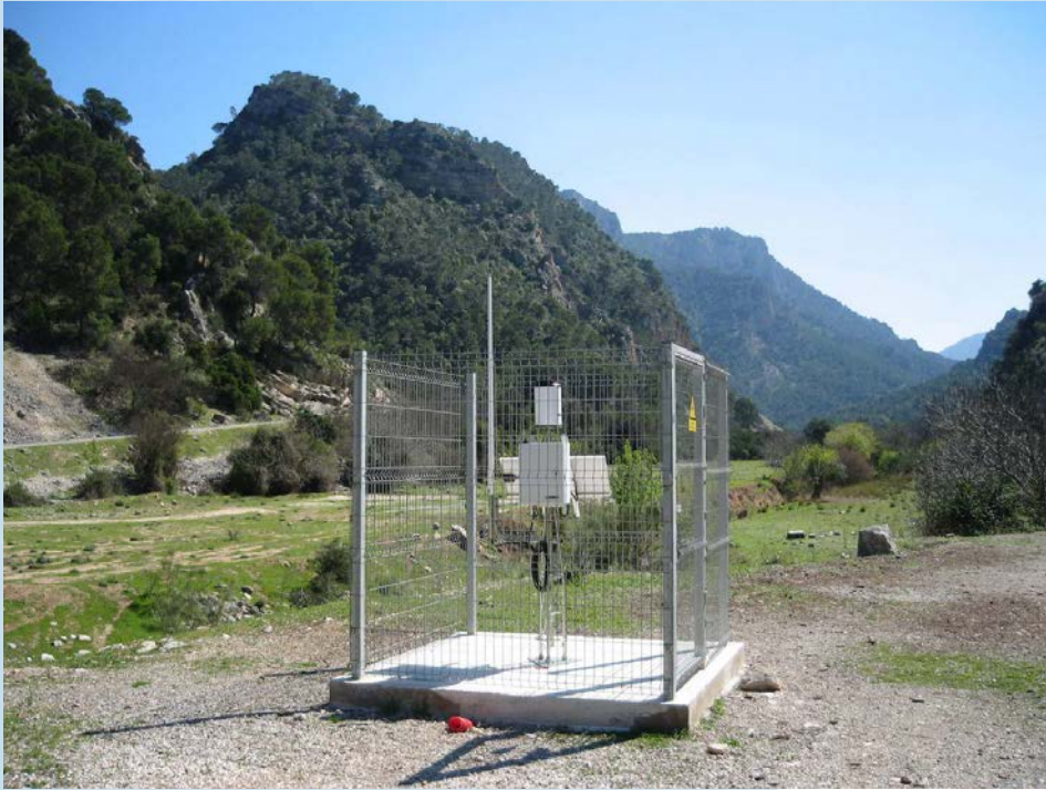
Remote Automatic Rainfall Measuring Station
